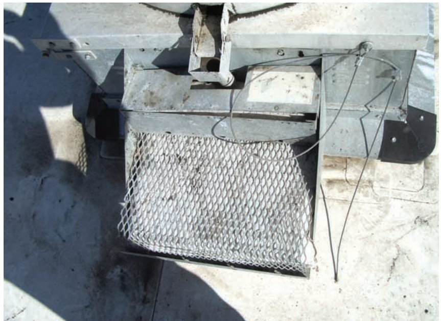
Applebee's Murrieta extractor with the new system, 6 months since prior cleaning. Notice there is no overflow 6 months after prior cleaning — the roof area around the extractor remains grease free.
